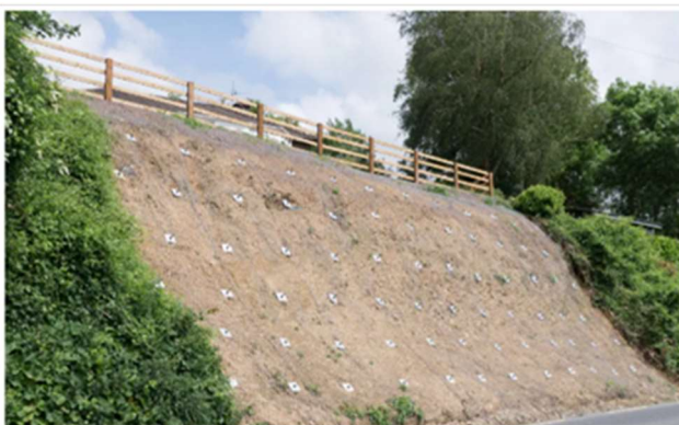
Figure 5-6 Typical Soil Nail / Anchor Installation
