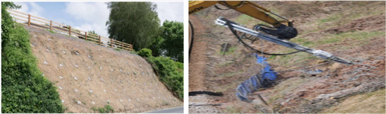
Figure 5-130 Example of Soil Nail Installation
