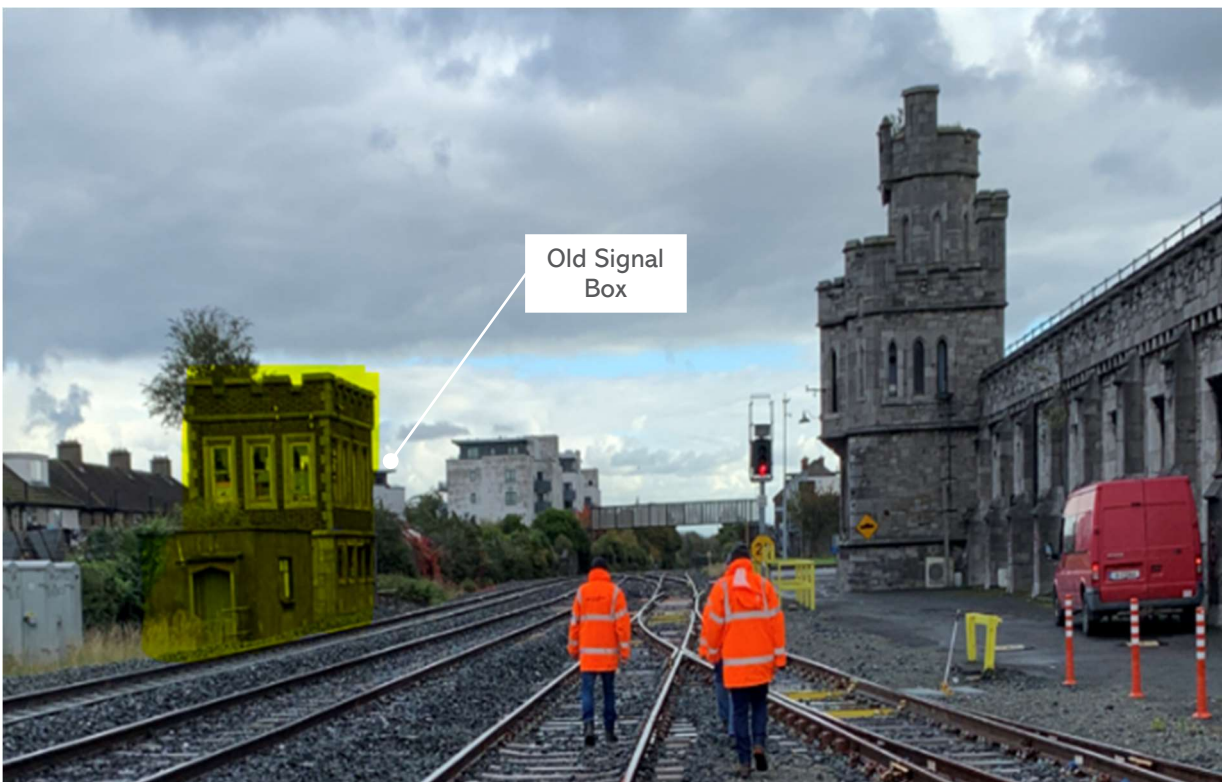
Figure 5-69 Old Signal Box to be Recorded and Removed (Highlighted in Yellow)
